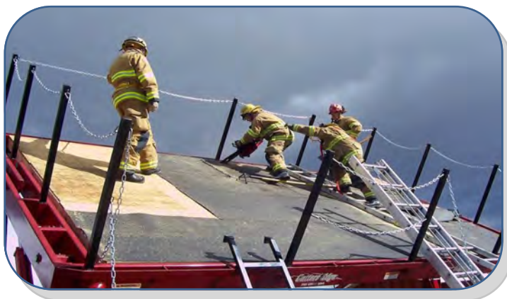
The new Dearborn Fire Training Academy will provide firefighters a controlled environment while giving them important practical experience, such as breaching a roof.
